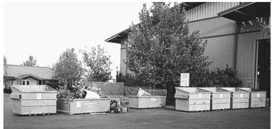
FIGURE 8.6 Example of drop-off center for the 24-h recovery of recyclables brought by community residents. Drop-off bins are located at entrance to MRF (see Figure 8.8).
