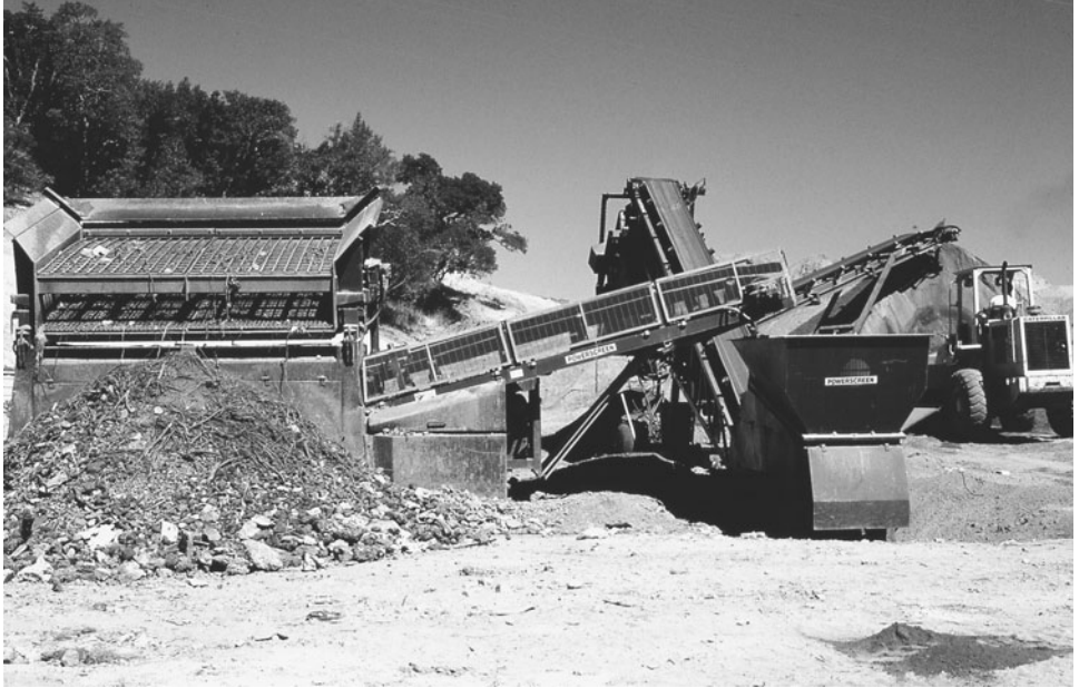
FIGURE 11D.4 Two-stage vibrating screen for the first-stage processing of excavated soil containing broken concrete, bricks, and tree roots. The screened soil from the first-stage screening is conveyed to a second, finer, set of screens for further processing. The final screen product is stockpiled in the background for reuse.
