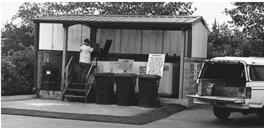
FIGURE 8.5 Drop-off facility for the recovery of used oil (note containers for the collection of used oil filters, and secondary containment berm in case of accidental spill).
