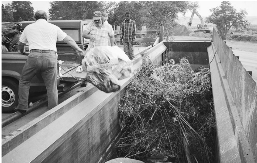
FIGURE 14.36 Small direct-load convenience transfer station located at landfill.
