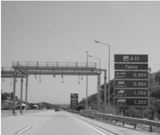
Figure 2. Free-flow tolling on A22 Portugal. (Reproduced with permission from Martial Chevreuil © Martial Chevreuil.)
