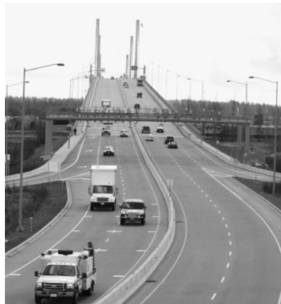
Figure 1. Golden Ears Bridge. (Reproduced by permission of Egis. © Egis.)
