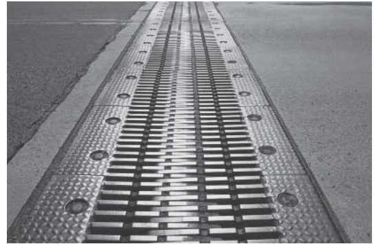
(b) Bridge expansion joint
