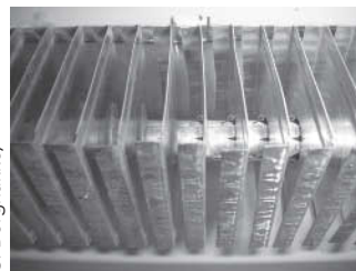
(b) Inside of a baseboard heater
