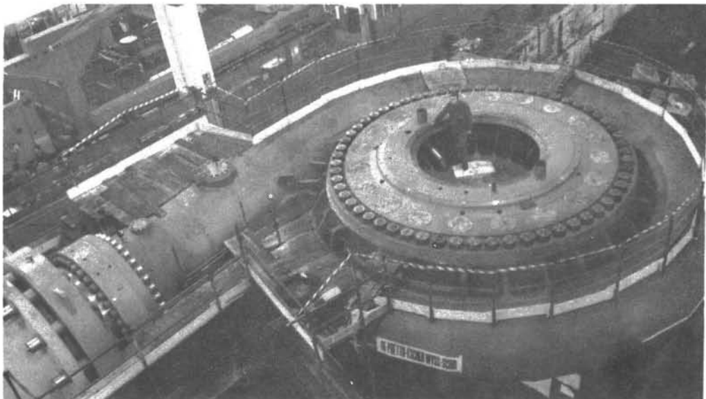
Fig. 6.2 Workshop pressure testing of spiral casing in Zurich, Switzerland.
