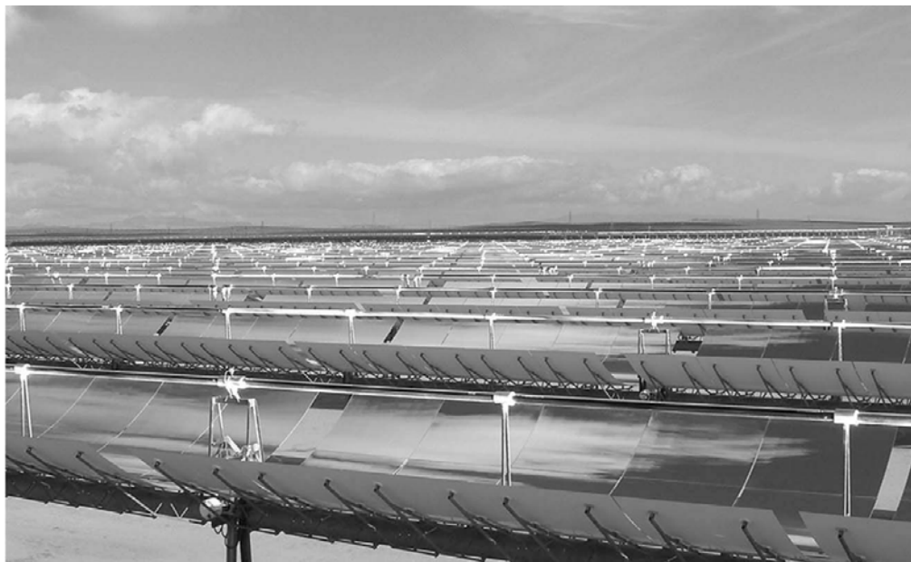
Figure 1: Parabolic solar trough collectors used to collect solar energy. The pipe located at the focal point of the receiver carries a heat transfer fluid.
