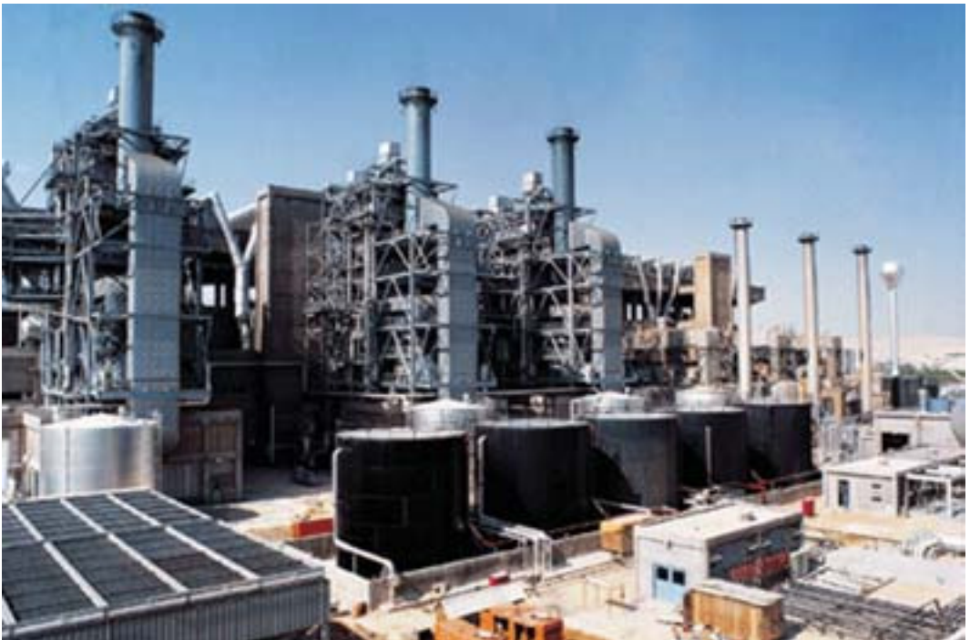
An overview of a thermal power station.
