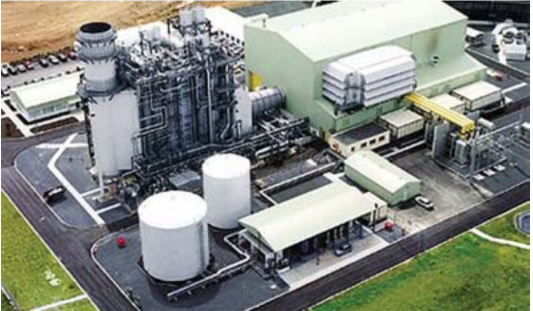
An overview of a combined cycle power plant. Governors are used in power plants to control the flow of working fluids.
