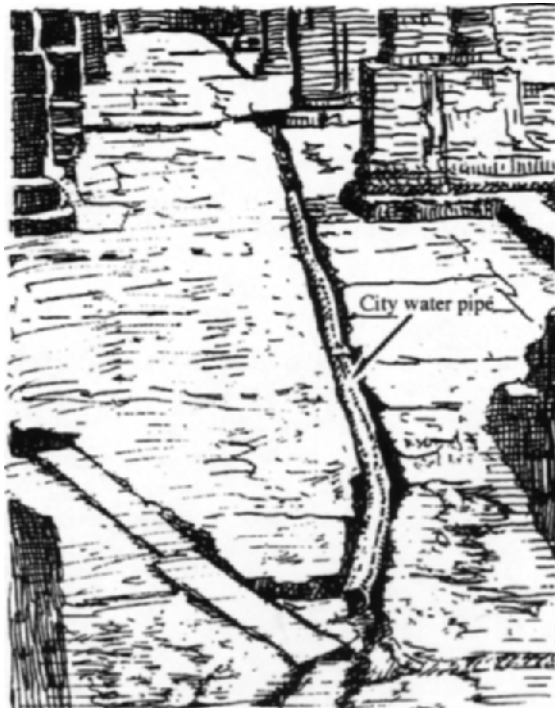
Lead city water pipe (Roman remains, Bath, England)
