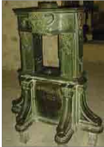
This screw press was made in 1735 and installed in the Segovia Mint to strike a new series of copper coins which began in 1772. This press is presently on display in the Alcazar castle of Segovia.
