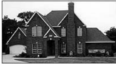
Fig. 2.42. This 3,000 sq. ft. house in Oklahoma City has a verified average electric bill of $60 per month using a geothermal heat pump.
