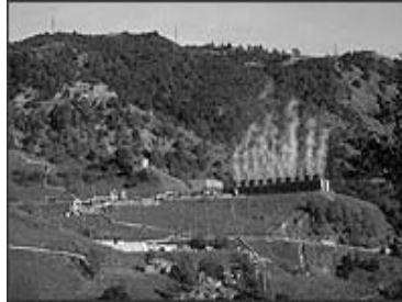
Fig. 2.33. A Geothermal Power Plant at the Geysers.
