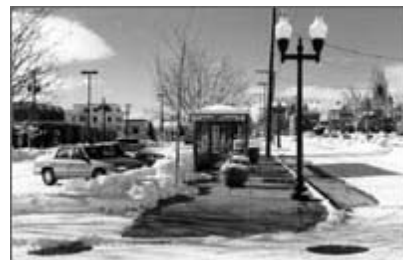
Fig. 2.40. Snow Melting on Sidewalks in Klamath Falls.
