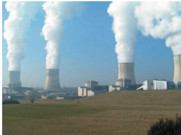
Fig. 18.4 A nuclear power plant. (Courtesy of R2 Controls)
