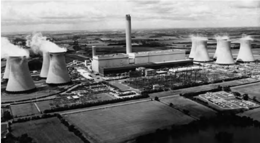
Fig. 15 Atmospheric cooling tower
