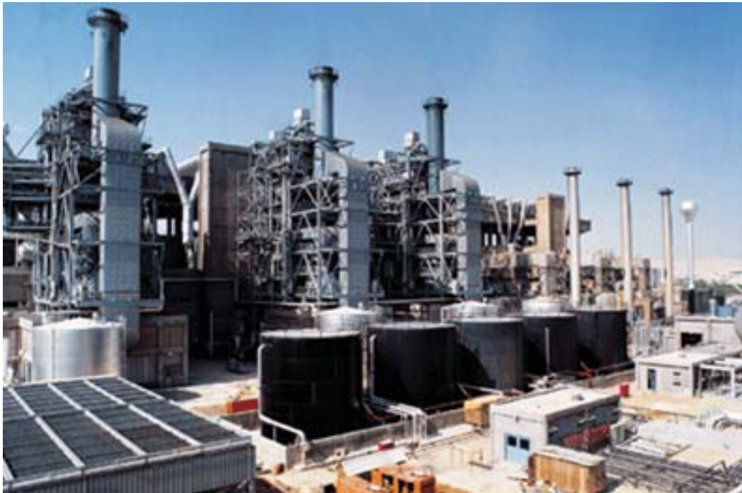
An overview of a thermal power station.
