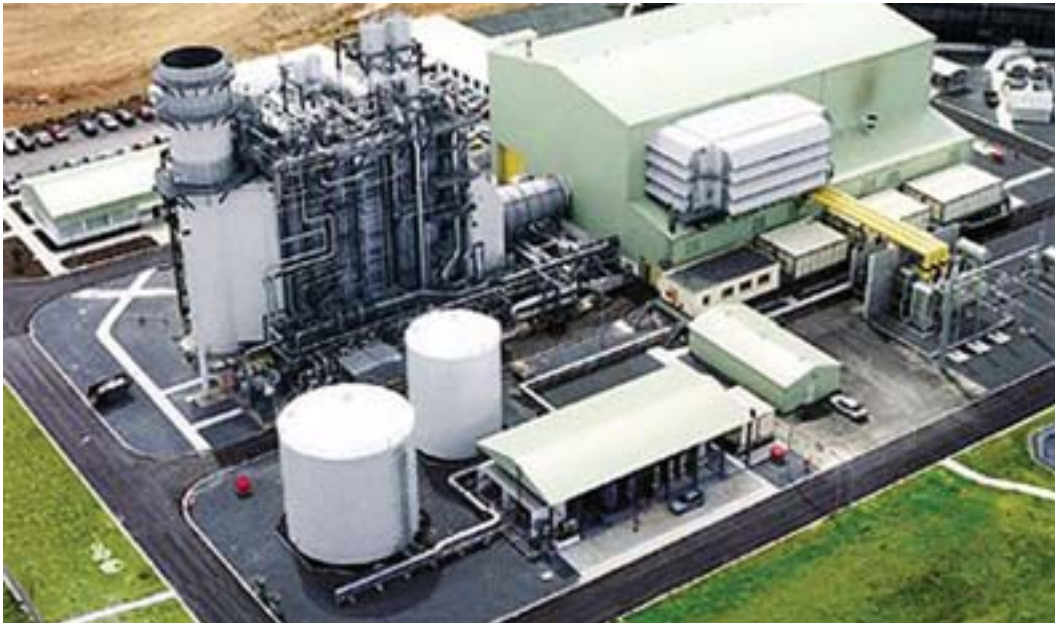
An overview of a combined cycle power plant. Governors are used in power plants to control the flow of working fluids.
