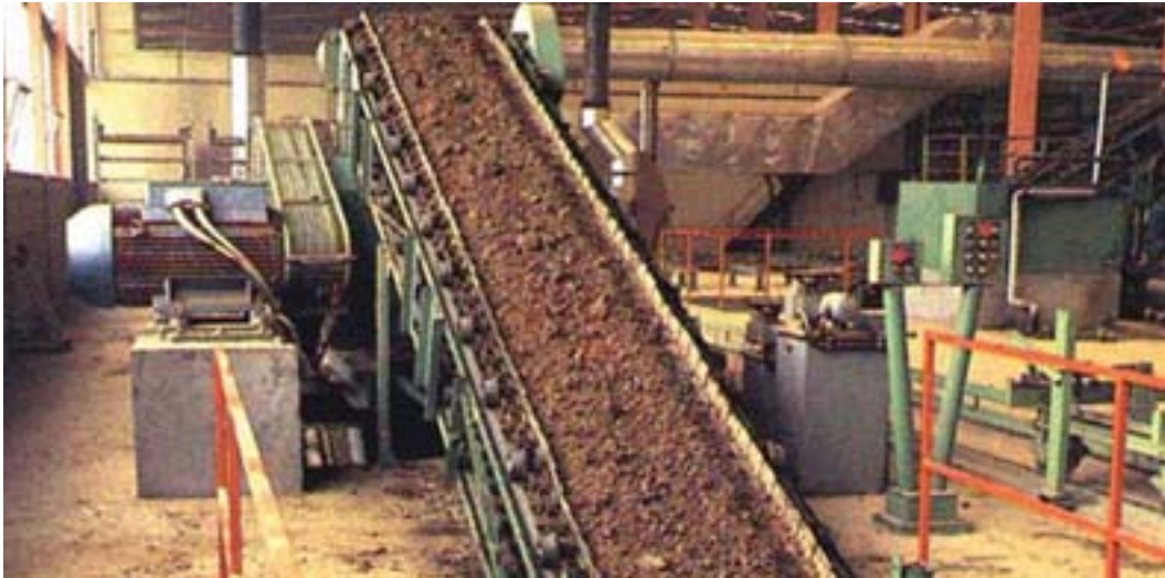
Material being moved via-belt conveyor.
