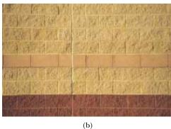
**Figure 19.6** (a) Thermal-expansion joints are used to separate sections of roadways on bridges. Without these joints, the surfaces would buckle due to thermal expansion on very hot days or crack due to contraction on very cold days. (b) The long, vertical joint is filled with a soft material that allows the wall to expand and contract as the temperature of the bricks changes.
