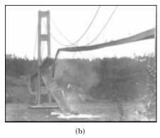
**Figure 13.23** (a) In 1940 turbulent winds set up torsional vibrations in the Tacoma Narrows Bridge, causing it to oscillate at a frequency near one of the natural frequencies of the bridge structure. (b) Once established, this resonance condition led to the bridge's collapse.
