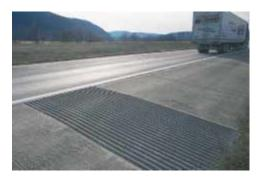
**Figure 18.13** Rumble strips along the side of a highway.
