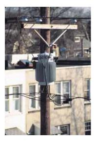
This cylindrical step-down transformer drops the voltage from 4 000 V to 220 V for delivery to a group of residences. (George Semple)
