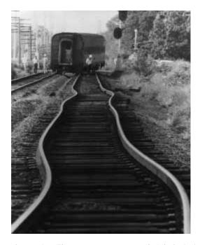
Thermal expansion: The extreme temperature of a July day in Asbury Park, NJ, caused these railroad tracks to buckle and derail the train in the distance. (AP/Wide World Photos)
