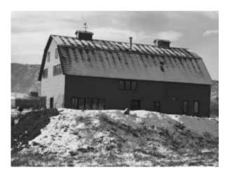
**Figure 020.10** Alternating pattern on a snow-covered roof.
