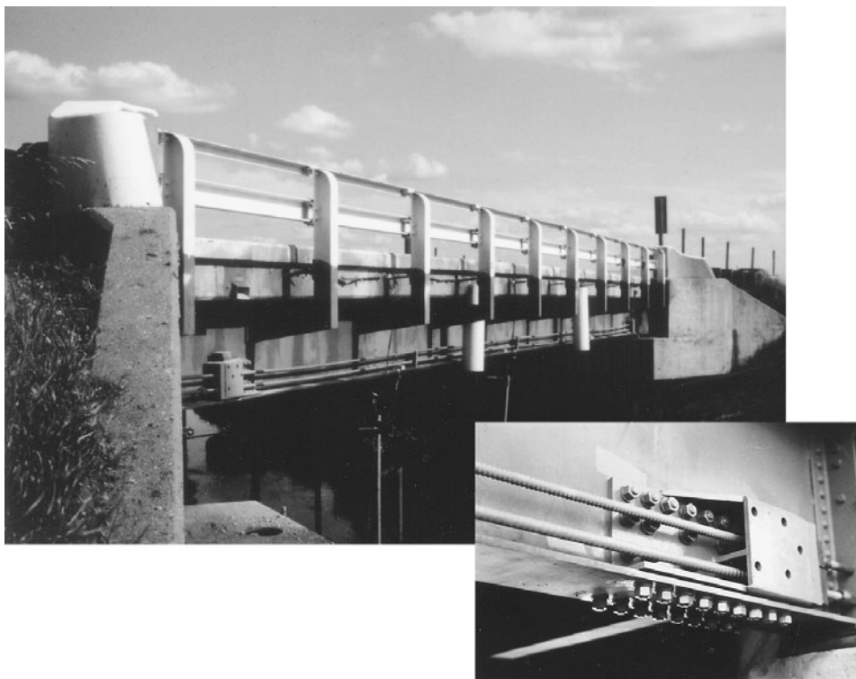
FIGURE 6.23 Single-span bridge strengthened by post-tensioning.
