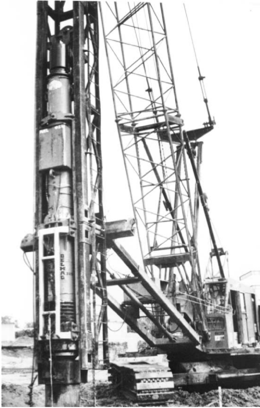
Fig. 7.19 Open-end, single-acting diesel hammer driving a pile.
