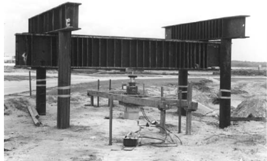
Fig. 7.24 Reaction piles used in static-load test on a pile.
