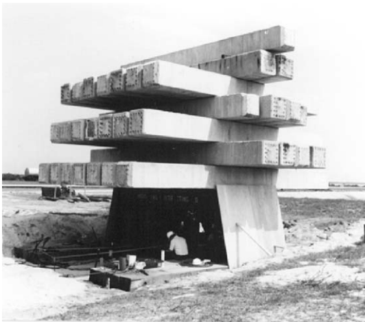
Fig. 7.23 Static-load test on a pile with dead weight as the reaction load.
