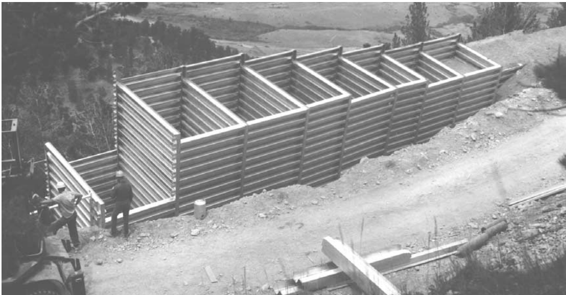
Fig. 10.26 Bin-type retaining wall of cold-formed steel.
