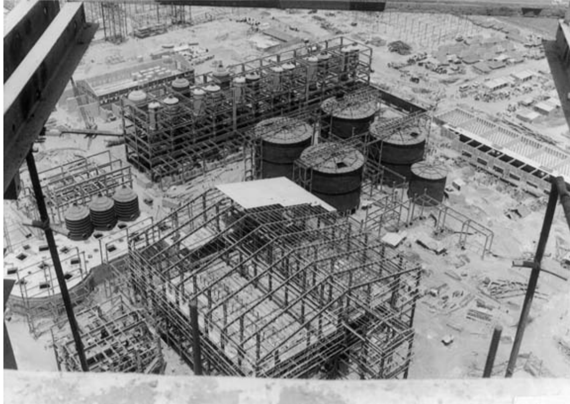
Fig. 10.11 Jacobson reaction system, 2500 tons per day P_2O_5 .
