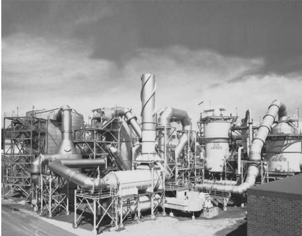
Fig. 14.10 Modern metallurgical sulfuric acid plant with view of preheating furnace in foreground. (Courtesy of Kennecott, Monsanto Enviro-Chem, and Manly Prim Photography)
