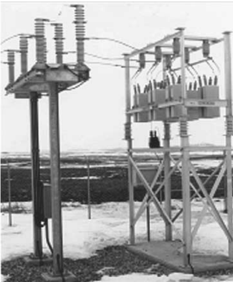
Figure 4.27 Synchronous closing capacitor switch. (Courtesy of Joslyn Hi-Voltage Corporation.)
