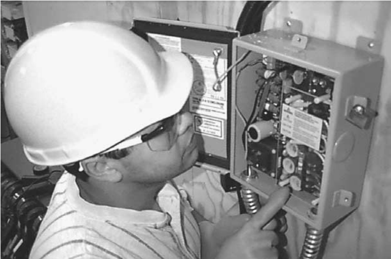
Figure 11.15 A low-cost power quality monitor that can page power quality engineers when disturbances occur.
