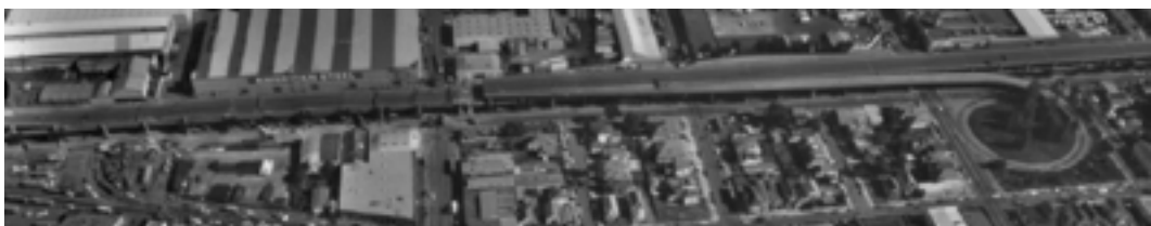
FIGURE 30.29 Aerial view of Cypress Street Viaduct showing collapse at north end (left) where the structure crossed over Bay mud, while the southern part (right), supported by dense sand, remained standing.
