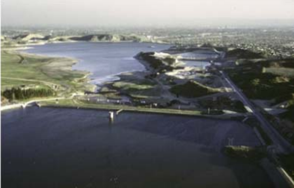
FIGURE 30.23 Aerial view of Lower San Fernando Dam and San Fernando Valley. (Courtesy of Steinbrugge Collection, Earthquake Engineering Research Center, University of California, Berkeley.)
