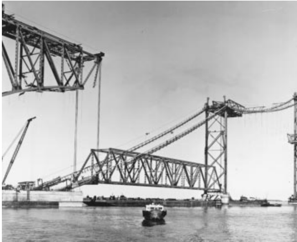
FIGURE 20.32: Erection of a truss span by hoisting, first Chesapeake Bay Bridge, Maryland, 1952. A 360-ft (110-m) truss span is floated into position on barges and picked clear using four sets of lifting falls. Suspension bridge deck is under construction at right. (Courtesy of Bethlehem Steel Corporation.)
