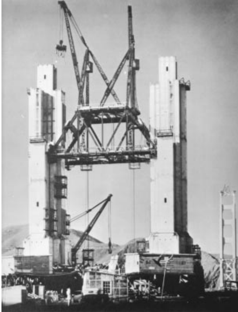
FIGURE 20.22: Erecting south tower of Golden Gate Bridge, San Francisco, 1935. A creeper traveler with two 90-ft (27-m) booms erects a tier of tower cells for each leg, then is jumped to the top of that tier and proceeds to erect the next tier. The tower legs are 90 ft (27 m) center-to-center and 690 ft (210 m) high. When the traveler completed the north tower (in background) it erected a Chicago boom on the west tower leg, which dismantled the creeper, erected tower-top bracing, and erected two small derricks (one shown) to service cable erection. Each tower contains 22,200 tons of steelwork.
