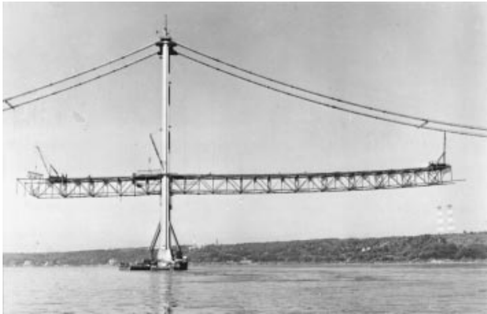
FIGURE 20.27: Erection of suspended deck steelwork, second Tacoma Narrows Bridge, Washington, 1950. The Chicago boom on the tower raises deck steelwork components to deck level, where they are transported to deck travelers by material cars. Each truss double panel is connected at top-chord level to previously erected trusses, and left open at bottom-chord level to permit temporary upward deck curvature, which results from the partial loading condition of the main suspension cables. The main span (at right) is 2800 ft (853 m), and side spans are 1100 ft (335 m). The stiffening trusses are 33 ft (10 m) deep and 60 ft (18 m) on centers. Tower-base kneebraces (see Figure 20.24) show clearly here.
