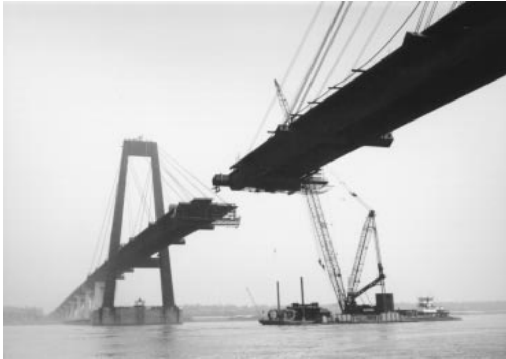
FIGURE 20.9: Cable-stayed orthotropic-steel-deck bridge over Mississippi River at Luling, La., 1982; view looking northeast. The main span is 1222 ft (372 m); the A-frame towers are 350 ft (107 m) high. A barge-mounted ringer derrick erected the main steelwork, using a 340-ft (104-m) boom with a 120-ft (37-m) jib to erect tower components weighing up to 183 tons, and using a shorter boom for deck components. Cable stays at the ends of projecting cross girders are permanent; others are temporary erection stays. Girder section 16-west of north portion of bridge, erected a few days previously, is projecting at left; companion girder section 16-east is on barge ready for erection (see Figure 20.10).
