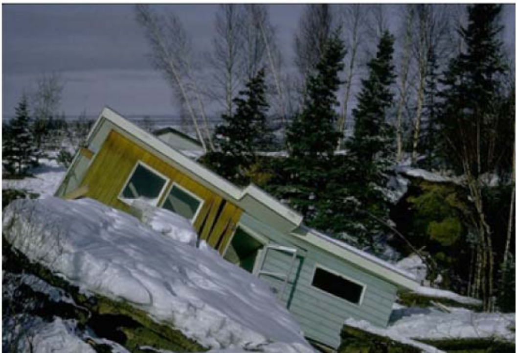
FIGURE 30.18 One of about 75 homes damaged as a result of the Turnagain Heights slide. (Courtesy of the Steinbrugge Collection, Earthquake Engineering Research Center, University of California, Berkeley.)
