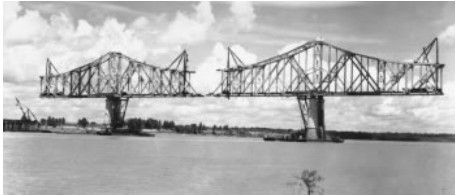
FIGURE 20.23: Balanced-cantilever erection, Governor O.K. Allen railway/highway cantilever bridge, Baton Rouge, La., 1939. First use of long balanced-cantilever erection in the U.S. On each pier 650 ft (198 m) of steelwork, about 4000 tons, was balanced on the 40-ft (12-m) base formed by a sloping falsework bent. The compression load at the top of the falsework bent was measured at frequent intervals and adjusted by positioning a counterweight car running at bottom-chord level. The main spans are 848-650-848 ft (258-198-258 m); 650 ft span shown. (Courtesy of Bethlehem Steel Corporation.)
