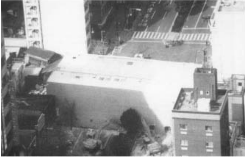
FIGURE 30.42 Eventual collapse of nine-story steel and reinforced-concrete (SRC) building after the Kobe earthquake. (Courtesy of NIST [9].)
