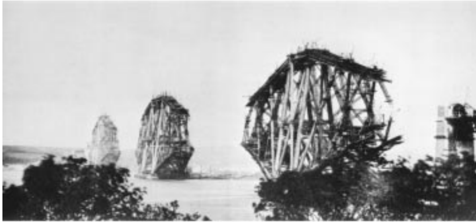
The massive cantilevers of the Forth bridge, shown under erection, were conceived in the shadow of the Tay bridge disaster.
