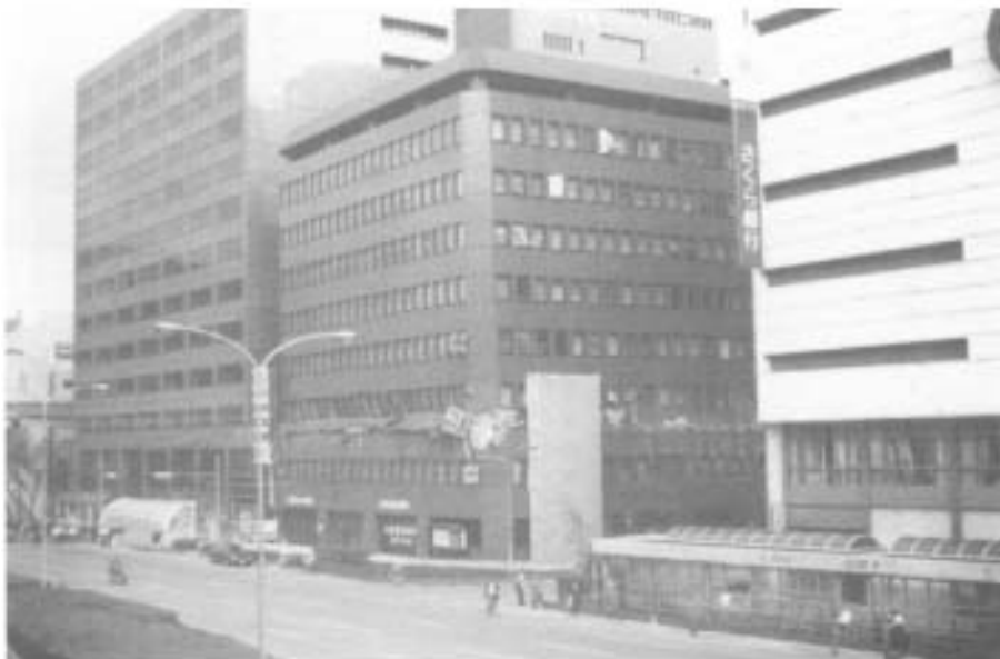
FIGURE 30.39 Ten-story steel and reinforced-concrete (SRC) building with third-floor collapse during the Kobe earthquake. (Courtesy of NIST [9].)
