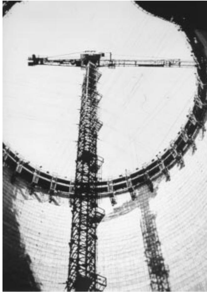
FIGURE 14.13: Attachments on shell wall.
