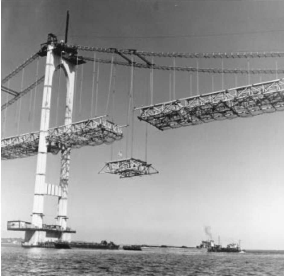
FIGURE 20.40: Suspended deck steelwork erection, the Newport Bridge suspension spans, Narragansett Bay, R.I., 1968. The closing mainspan deck section is being raised into position by two cable travelers, each made up of a pair of 36-in. (0.91-m) wide-flange rolled beams that ride the cables on wooden wheels. The closing section is 40-1/2 ft (12 m) long at top-chord level, 66 ft (20 m) wide and 16 ft (5 m) deep, and weighs about 140 tons. (Courtesy of Bethlehem Steel Corporation.)
