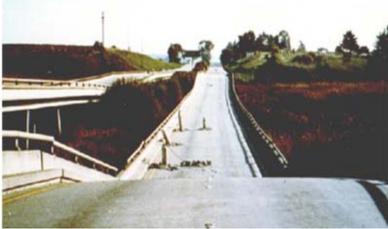
FIGURE 30.26 Piles penetrating the bridge deck.
