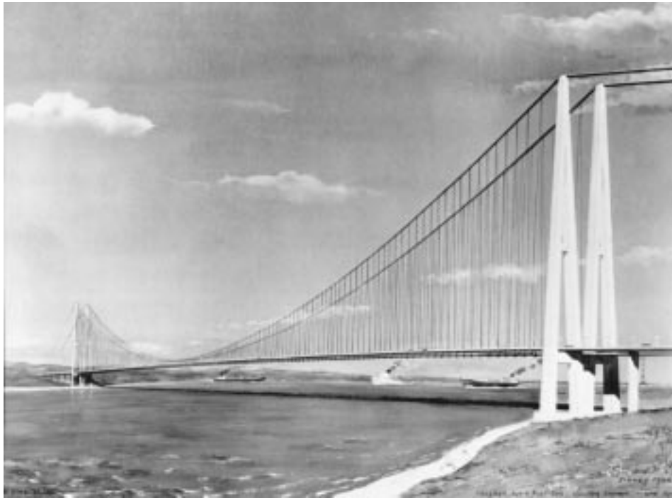
FIGURE 20.47: Artist's rendering of proposed Messina Strait suspension bridge, Italy. The Messina Strait crossing has been under discussion since about 1850, under investigation since about 1950, and under active design since about 1980. The enormous bridge shown would connect Sicily to mainland Italy with a single span of 10,827 ft (3300 m). Towers are 1250 ft (380 m) high. The bridge construction problems for such a span will be tremendously challenging. (Courtesy of Stretto di Messina, S.p.A.)
