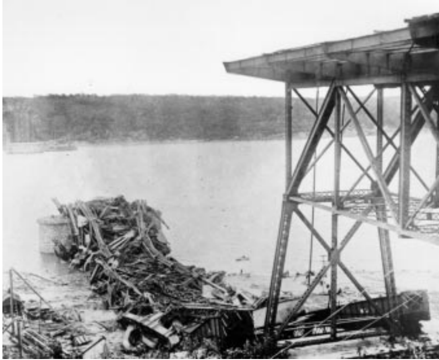
FIGURE 20.12: Wreckage of south anchor span of first Quebec railway cantilever bridge, 1907. View looking north from south shore a few days after collapse of 29 August 1907, the worst disaster in the history of bridge construction. About 20,000 tons of steelwork fell into the St. Lawrence River, and 75 workmen lost their lives.
