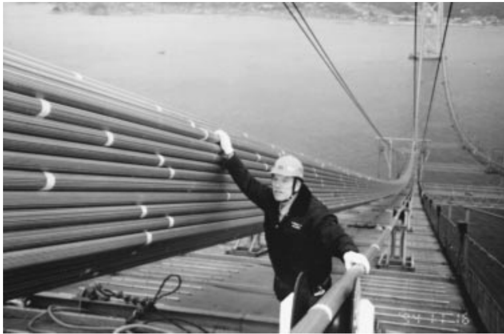
FIGURE 20.46: Parallel-wire-strand main cable, Akashi Kaikyo suspension bridge, Kobe, Japan, 1994. The main span is 6529 ft (1990 m), by far the world's longest. The PWS at right is being towed across the spans, supported on rollers. The completed cable is made up of 290 PWS, making a total of 36,830 wires, and has a diameter of 44.2 in. (1122 mm) following compaction—the largest bridge cables built to date. Each 127-wire PWS is about 2-3/8 in. (60 mm) in diameter. (Courtesy of Nippon Steel—Kobe Steel.)
