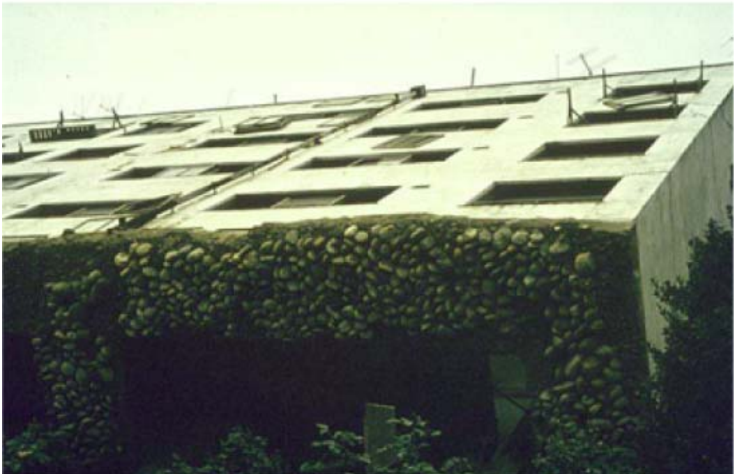
FIGURE 30.5 Liquefaction-caused building failure in Niigata, Japan. (Photograph by Joseph Penzien and courtesy of Steinbrugge Collection, Earthquake Engineering Research Center, University of California, Berkeley.)
