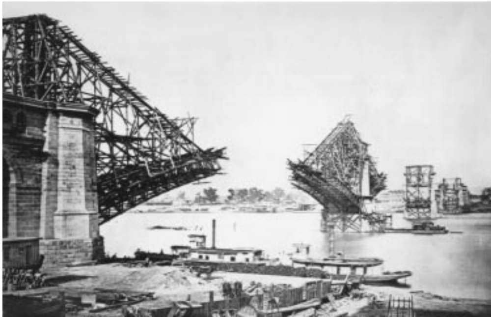
FIGURE 20.15: Eads Bridge across the Mississippi River, St. Louis, Mo., 1873. The first important metal arch bridge in the U.S., supported by four planes of hingeless trussed arches having chrome-steel tubular chords. Spans are 502-520-502 ft (153-158-153 m). During erection, arch ribs were tied back by cables passing over temporary towers built on the piers. Arch ribs were packed in ice to effect closure.
