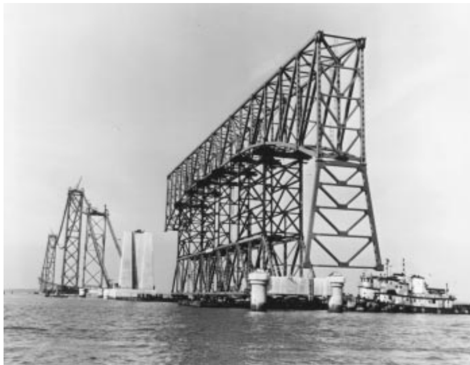
FIGURE 20.31: Floating-in erection of a truss span, first Chesapeake Bay Bridge, Maryland, 1952. A 480-ft (146-m) truss span, weighing 850 tons, supported on falsework consisting of a permanent deck-truss span along with temporary members, is being floated-in for landing onto its piers. Suspension bridge cables are under construction in background. (Courtesy of Bethlehem Steel Corporation.)
