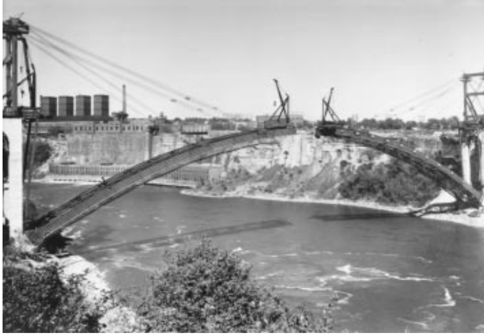
FIGURE 20.2: Erection of arch ribs, Rainbow Bridge, Niagara Falls, New York, 1941. Bridge span is 950 ft (290 m), with rise of 150 ft (46 m); box ribs are 3 \times 12 ft ( 0.91 \times 3.66 m). Tiebacks were attached starting at the end of the third tier and jumped forward as erection progressed (see Figure 20.3). Much permanent steelwork was used in tieback bents. Derricks on approaches load steelwork on material cars that travel up arch ribs. Travelers are shown erecting last full-length arch-rib sections, leaving only the short, closing crown sections to be erected. Canada is at right, the U.S. at left. (Courtesy of Bethlehem Steel Corporation.)
