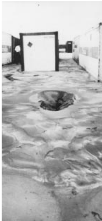
FIGURE 5.31: Photograph of sand boils.
