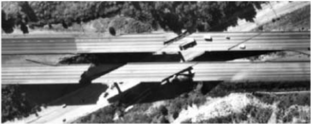
FIGURE 30.43 Damage to Gavin Canyon Undercrossing during the 1995 Northridge earthquake.
