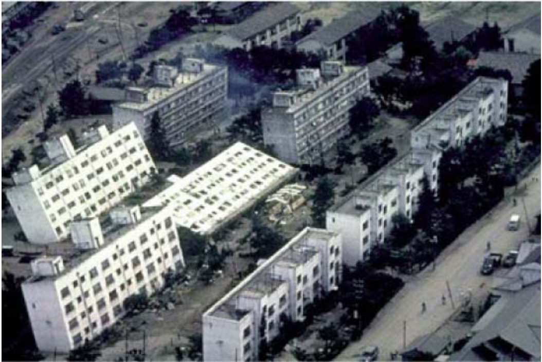
FIGURE 30.4 Liquefaction-caused building failure in Niigata, Japan. (Photograph by Joseph Penzien and courtesy of Steinbrugge Collection, Earthquake Engineering Research Center, University of California, Berkeley.)
