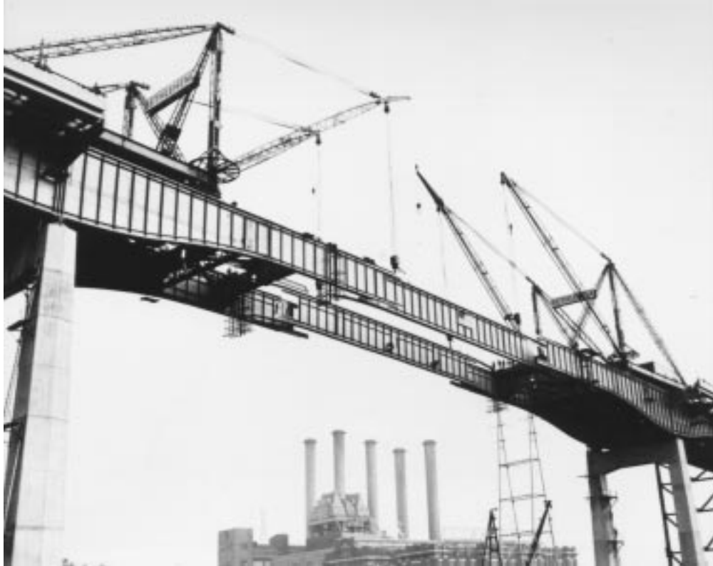
FIGURE 20.29: Erecting closing girder sections of Passaic River Bridge, New Jersey Turnpike, 1951. Huge double-boom travelers, each weighing 270 tons, erect closing plate girders of the 375-ft (114-m) main span. The closing girders are 14 ft (4.3 m) deep and 115 ft (35 m) long and weigh 146 tons each. Sidewise entry was required (as shown) because of long projecting splice material. Longitudinal motion was provided at one pier, where girders were jacked to effect closure. Closing girders were laterally stable without floor steel fill-in, such that derrick falls could be released immediately. (Courtesy of Bethlehem Steel Corporation.)
