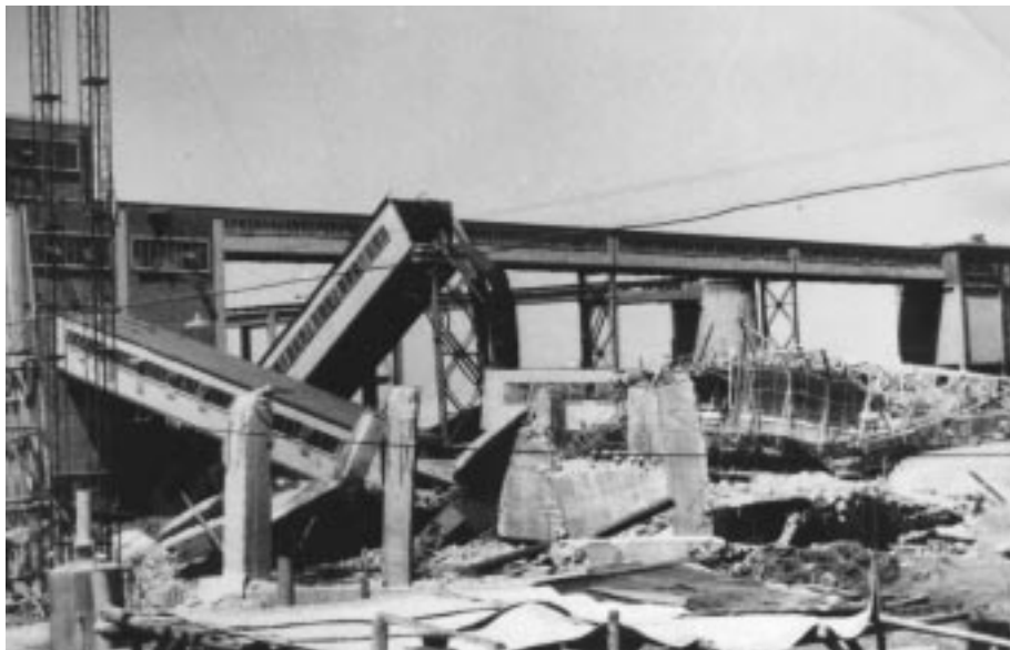
FIGURE 16.1: Collapsed elevated steel conveyor at Lujiatuo Mine following the 1976 Tangshan earthquake in China. (From California Institute of Technology, The Greater Tangshan Earthquake , California, 1996. With permission.)
