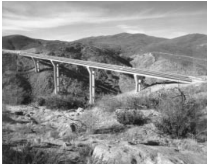
FIGURE 10.16 Pine Valley Bridge, California. Construction completed. (From California Department of Transportation. With permission.)
