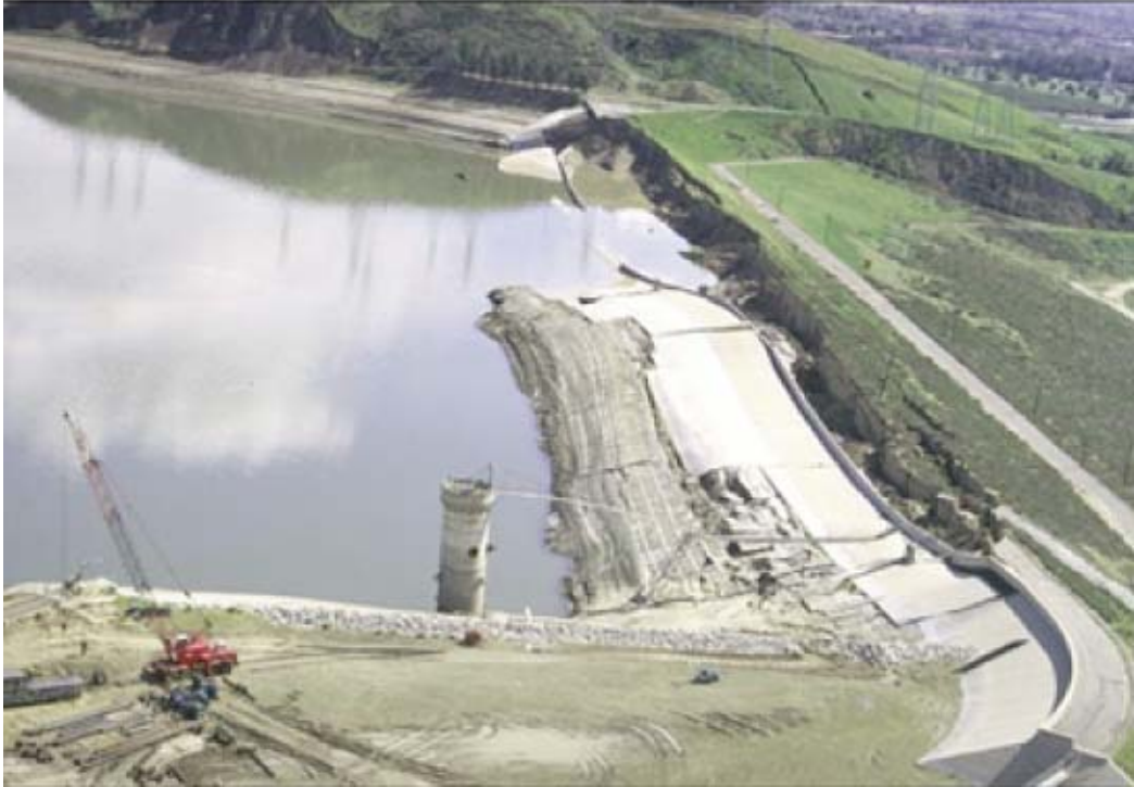
FIGURE 30.21 Damage to the Lower San Fernando Dam. (Courtesy of Steinbrugge Collection, Earthquake Engineering Research Center, University of California, Berkeley.)
