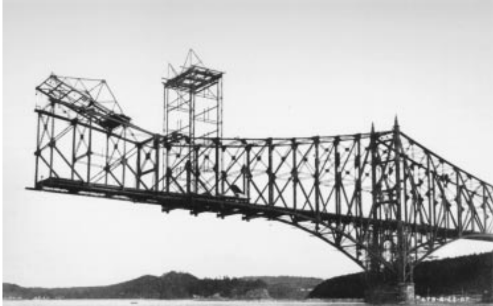
FIGURE 20.11: First Quebec railway cantilever bridge, 23 August 1907. Cantilever erection of south main span, 6 days before collapse. The tower traveler erected the anchor span (on falsework) and then the cantilever arm; then erected the top-chord traveler, which is shown erecting suspended span at end of cantilever arm. The main span of 1800 ft (549 m) was the world's longest of any type. The sidespan bottom chords second from pier (arrow) failed in compression because latticing connecting chord corner angles was deficient under secondary bending conditions.
