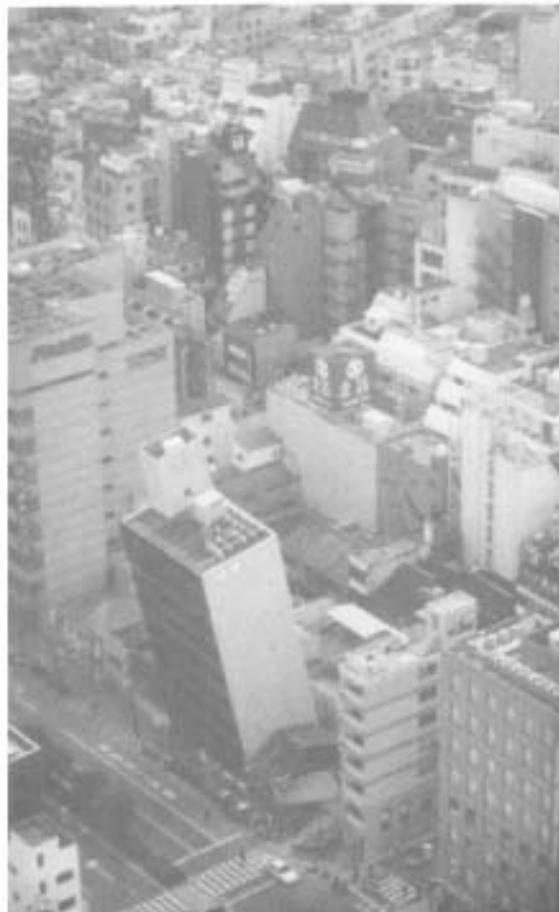
FIGURE 30.41 Nine-story steel and reinforced-concrete (SRC) building immediately after the 1995 Kobe earthquake. (Courtesy of NIST [9].)
