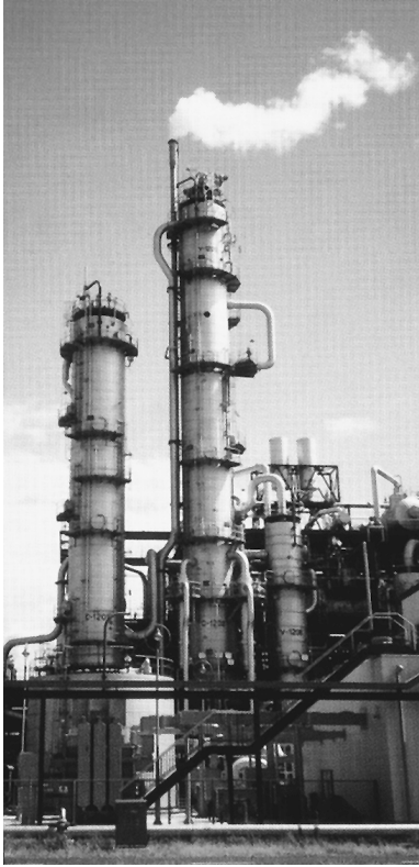
Fig. 6a. Distillation column (courtesy of Eickmeyer and Assoc.)
