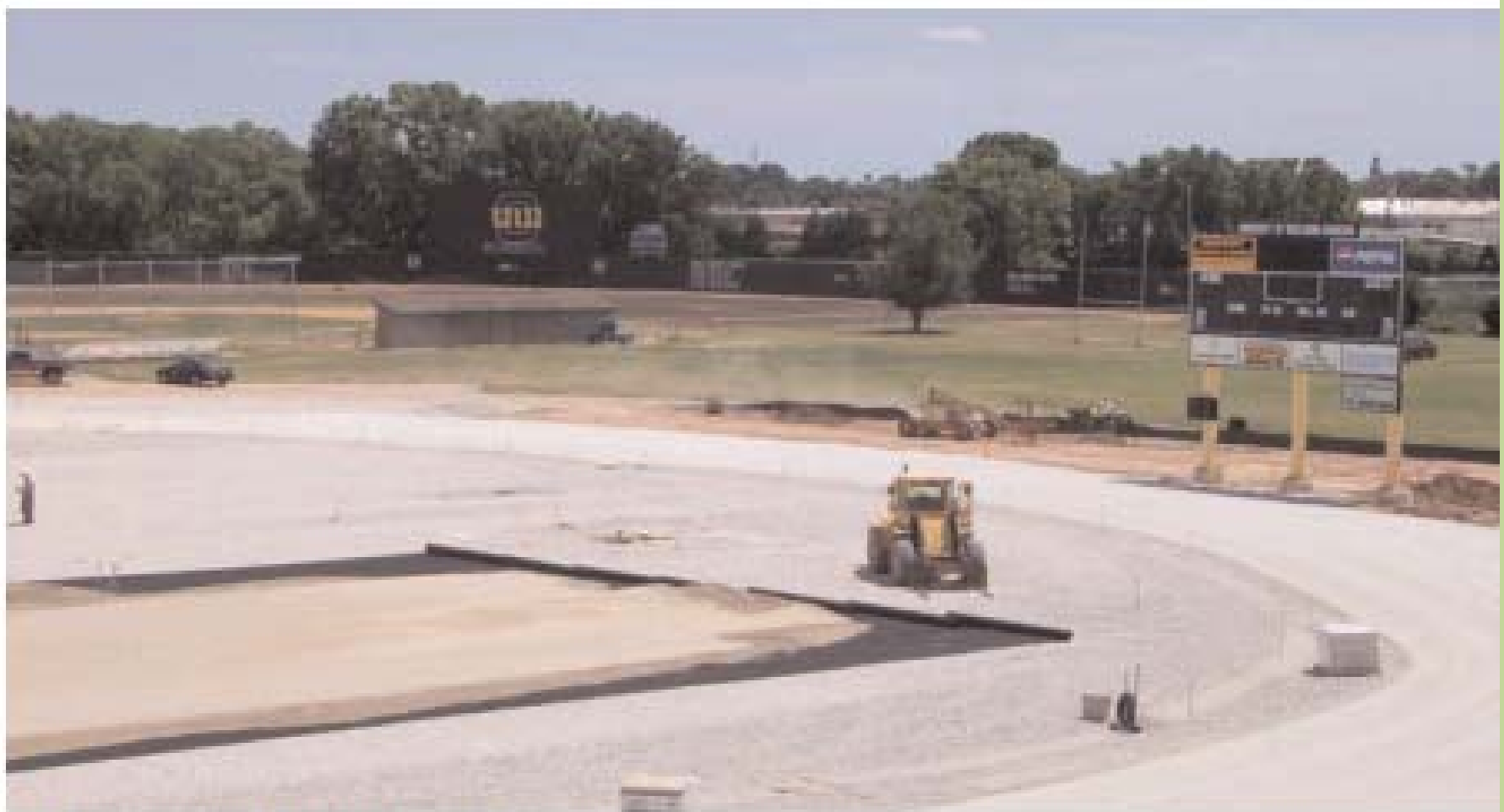
Installation of Mirafi ® FW402 geotextile.
