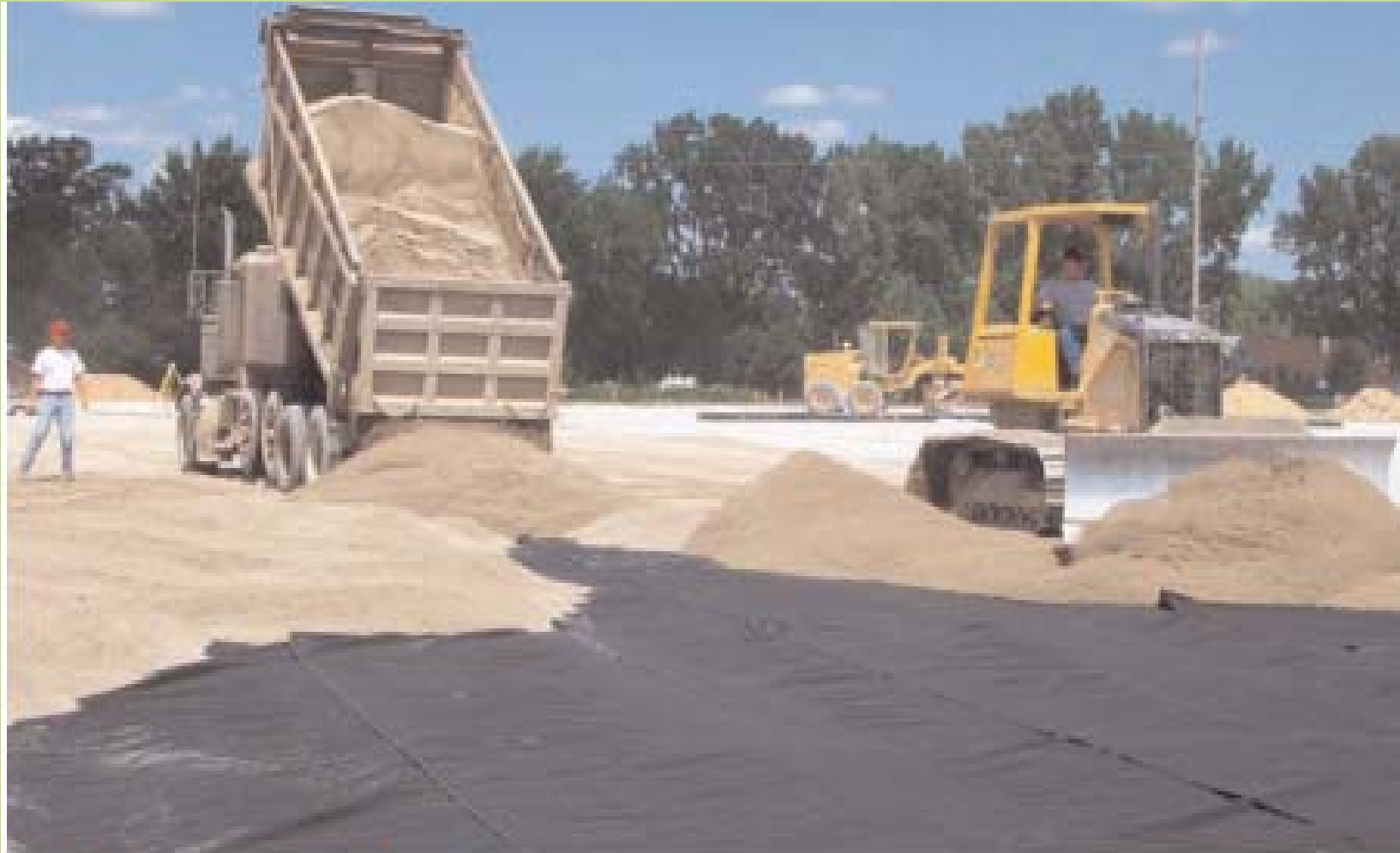
Backfill deployment on Mirafi ® FW402 geotextile.
