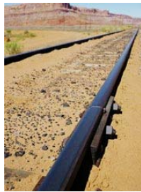
Loosening of side plates at rail joint
