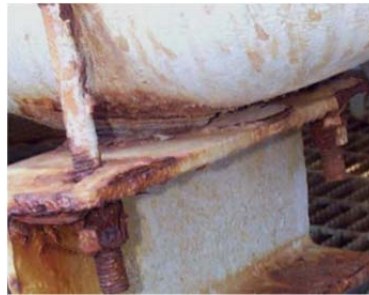
Corrosion at the corner of water Tank
