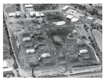
**FIGURE 19.8** The Exolon plant in Hennepin, IL. This plant is one of the newest SiC facilities in the world, producing both high-quality metallurgical and crystalline SiC annually. It is North America's only manufacturer of SiC. The plant features 16 furnaces operating off of four transformers.
