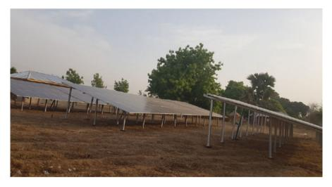
**Fig. 11.11** PV modules like these for a mini-grid in Angwan Rina, Nigeria, are often mounted on a rack to obtain the desired tilt (courtesy of GVE Projects)
