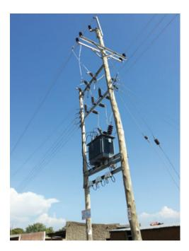
**Fig. 3.7** Pole-mounted three-phase distribution transformer in Kenya (courtesy of author)
