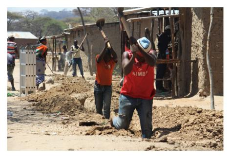
Fig. 12.9 Trenches being dug for underground distribution (courtesy of PowerGen)
