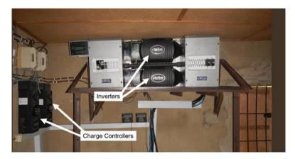
Fig. 9.31 A pair of inverters provide AC to a mini-grid in Nigeria (courtesy GVE Projects)
