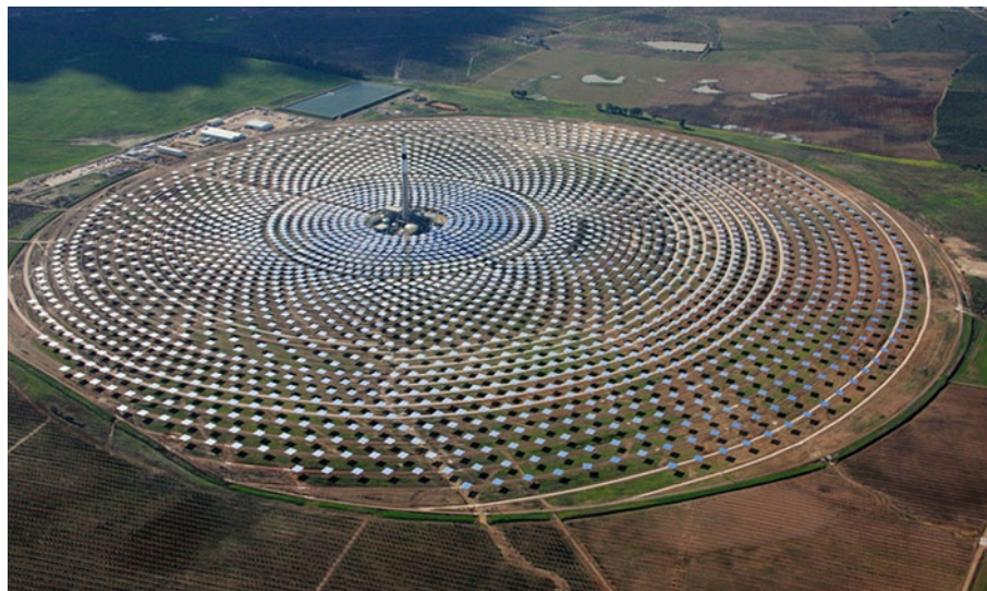
Figure 10.92 Gemasolar power station close to Sevilla. 2650 mirrors reflect the sun light onto a tower where a salt solution is heated. It will deliver electric energy of 110 GWh per year. (Torresol Energy Investment S.A.)
