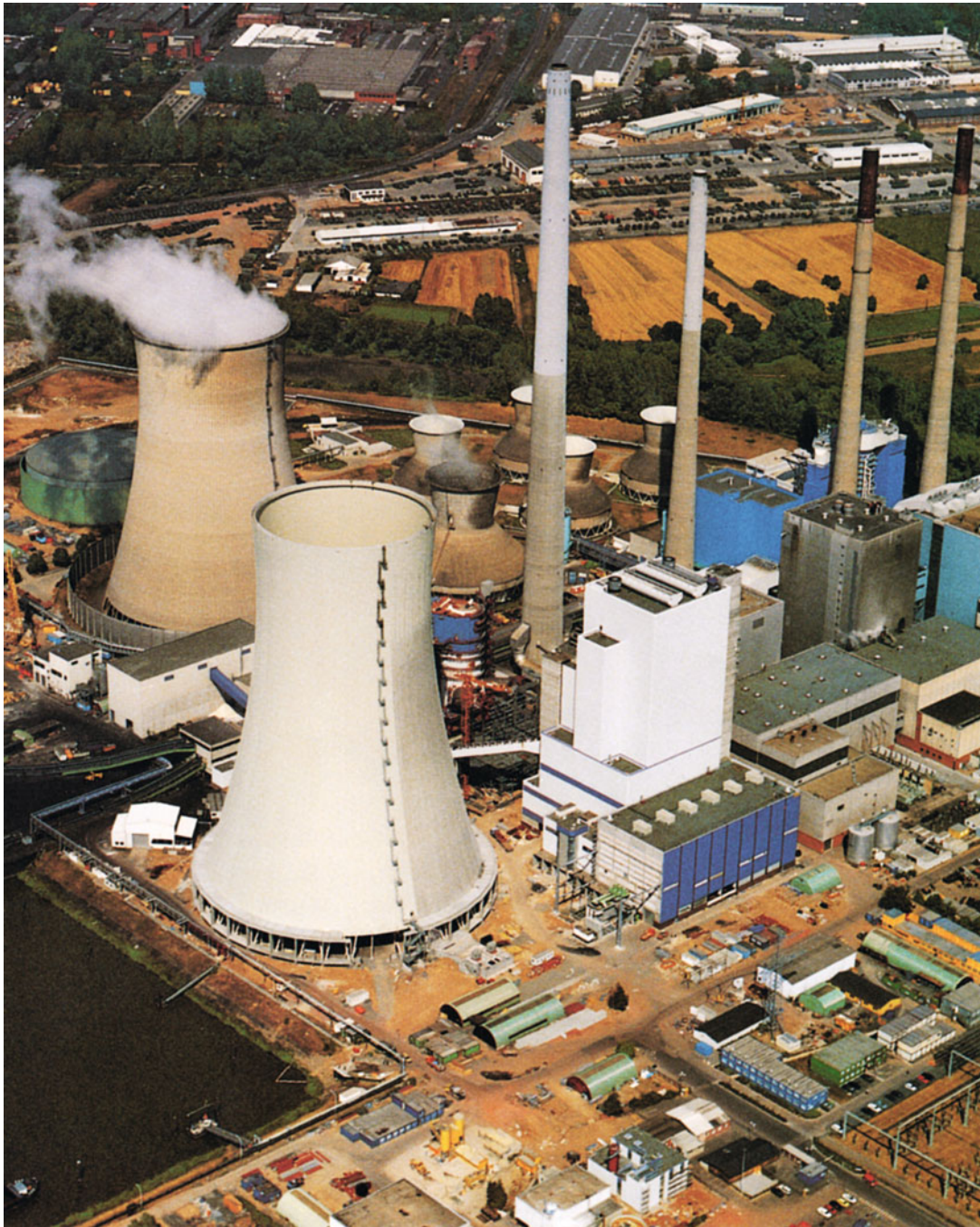
Figure 10.83 Cooling towers of the coal power plant Staudinger. The plant delivers 500 MW electric power and 300 MW heat power. It reaches an efficiency of 42.5% (With kind permission of Preußen Elektra AG, Hannover)
