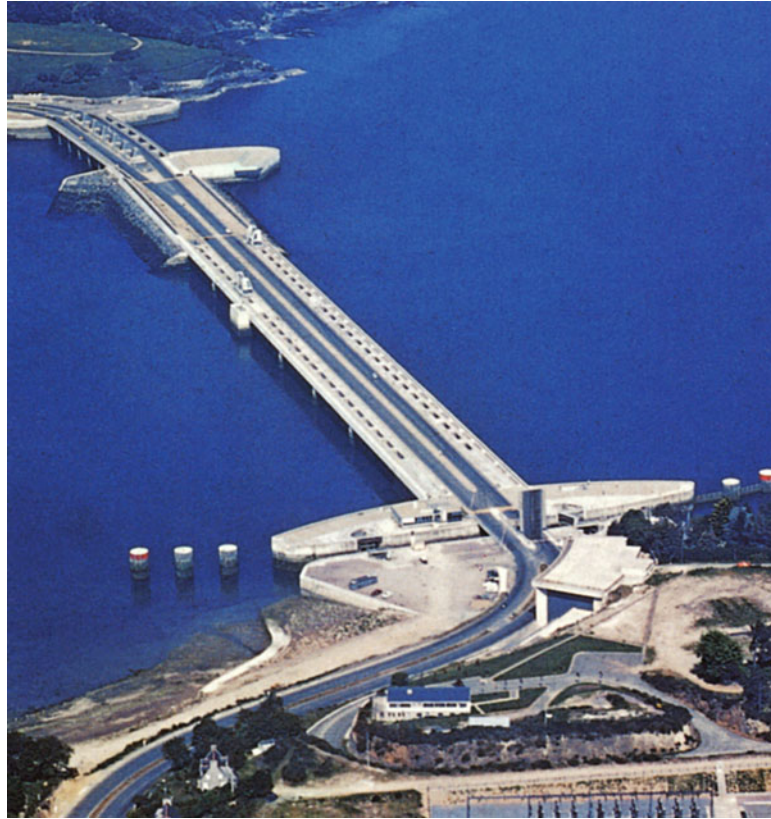
Figure 10.86 Tidal Power Station St.Malo. Aerial view of the power station in the estuary of the river Rance in France. Here the tidal amplitude is about 8 m (see Sect. 6.6). With kind permission © Foto dpa
