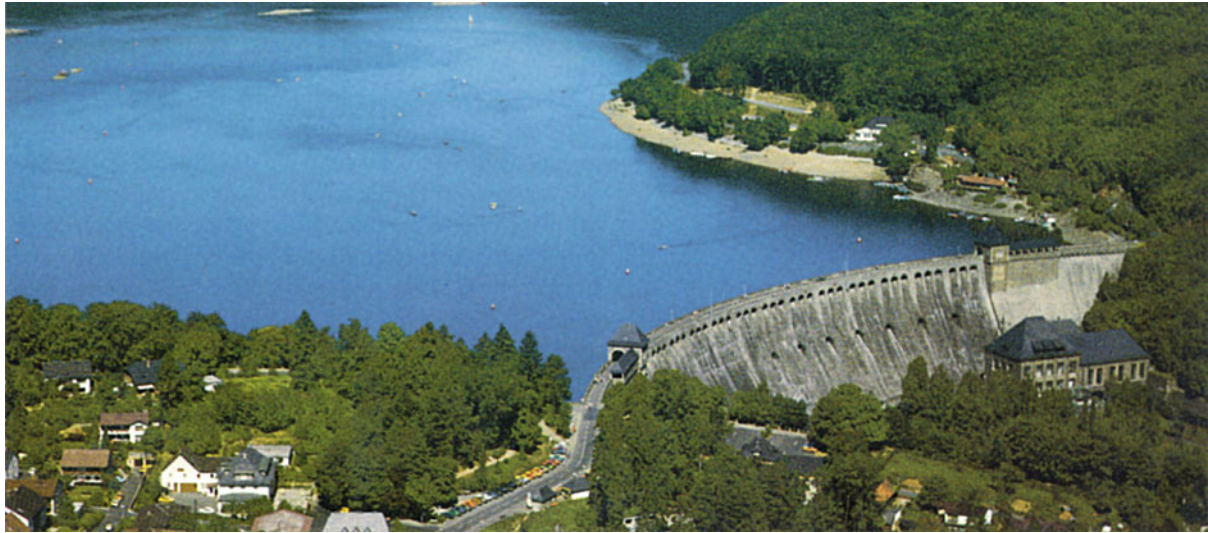
Figure 6.26 River dam of the river Eder, Germany. The bending of the dam towards the water side conducts part of the water pressure against the mountain sides (see Sect. 6.3). With kind permission of Cramers Kunstverlag, Dortmund
